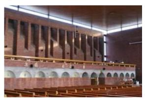
Above are the light chimneys from St Brides East Kilbride which are similar to the light chimneys on the eastern wall of St Patrick's which allow diffuse light to fall into the gallery area from the concealed window above. Note also the similarities of the wooden benches.
