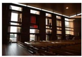
Above is the drawing of the West facing window at the rear of St Paul's Glenrothes the first modernist design by MacMillan and Metzstien. It bears remarkable similarity to the design of the western wall at St Patrick's in its use of thick horizontal elements and thin vertical elements.
