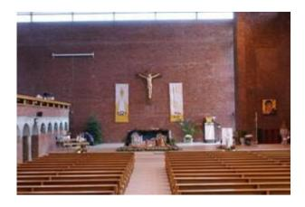
Post 1999/2000 restoration works. The same view of the southern elevation as in the black and white plate above. Significant improvement to the white efflorescence staining on the sanctuary wall is clear – although not removed entirely. The above picture is dated Dec 2008.
